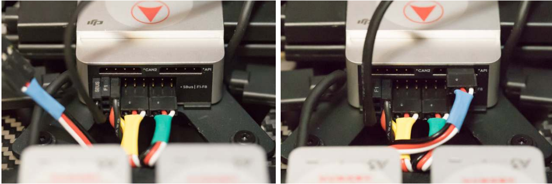
Figure 102: Three connectors installed.
