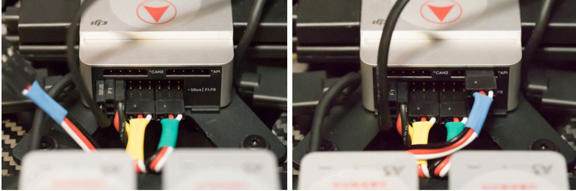
Figure 127: Three connectors installed.
