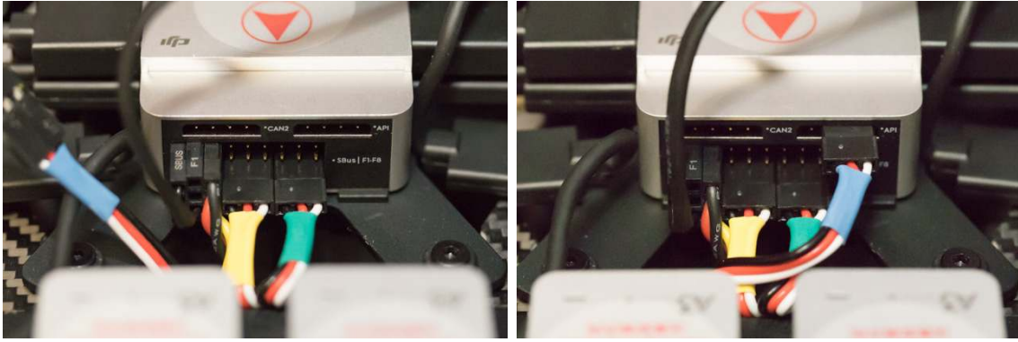
Figure 103: Three connectors installed.
